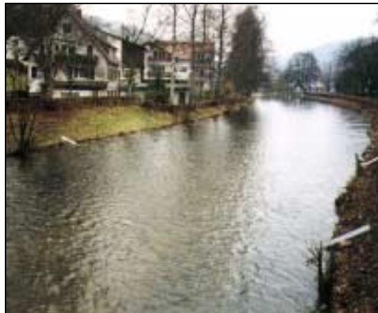
Picture 1: An ultrasonic flowmeter in a water course with moving current
